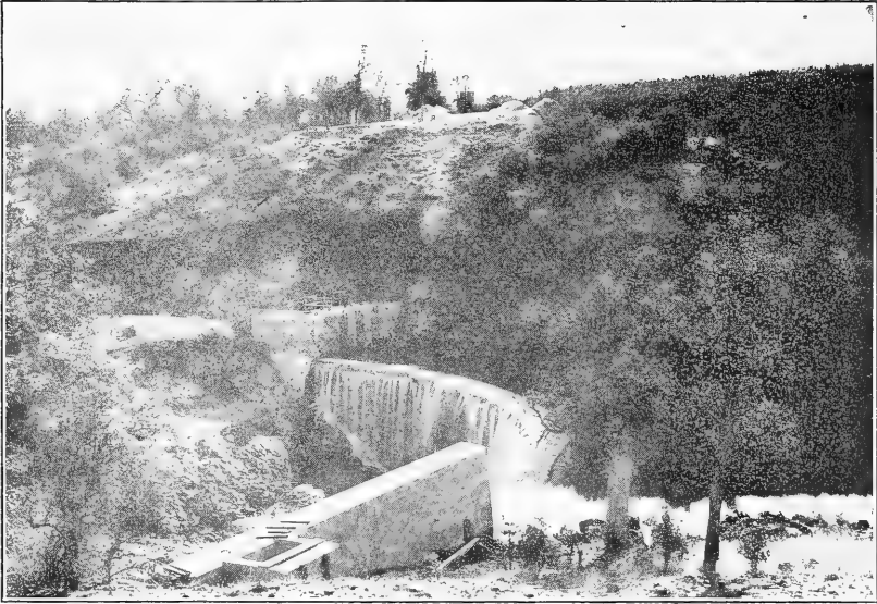
FIG. 1.—HEADWORKS, EAST PARK SUPPLY CANAL, ORLAND PROJECT, CALIFORNIA. Shows diversion of part of waters of Big Stoney Creek into East Park Reservoir. Note gate control of supply.
